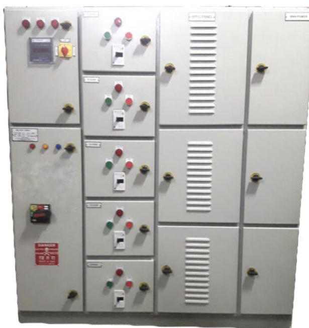
**BNN POWER Automatic Power Factor Correction System** is unique with its customized design, based on the Load Study conducted on site with Power Quality analyzer with recording. Electrical loads such as motors can cause electrical systems to be very inductive, which results in vary 'lagging power factor' whereas loads like UPS can cause Electrical load to be capacitive, which result in 'leading power factor' we consider both to maintain  $KWH=KVAH$ .
